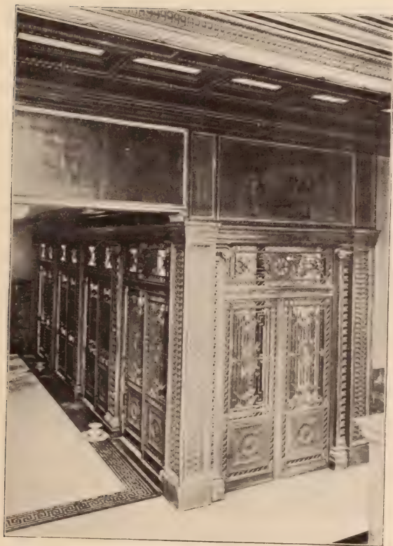
PASSENGER ELEVATOR ENCLOSURE, CONSTABLE BUILDING. Executed by Hecla Iron Works.
